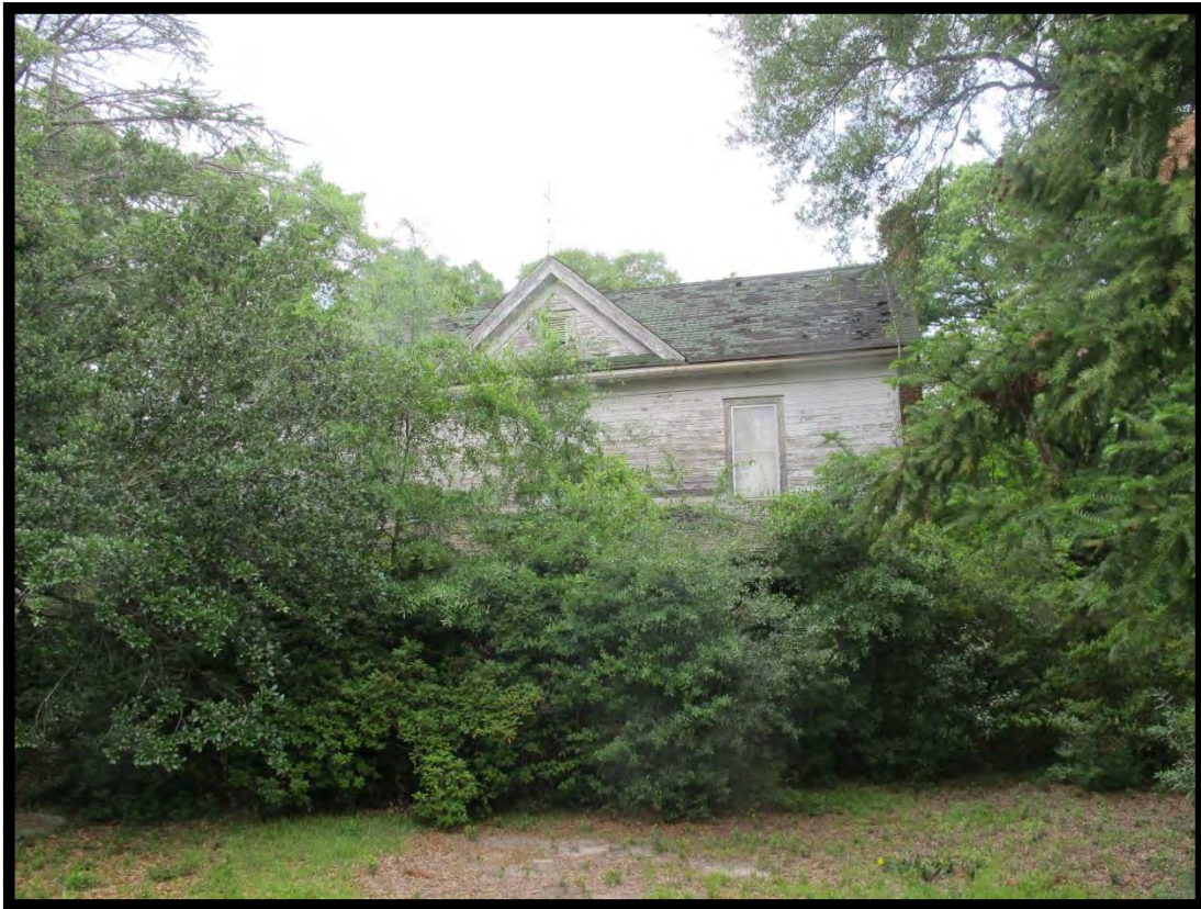
Figure 48: Ritter House, Looking Northwest.
