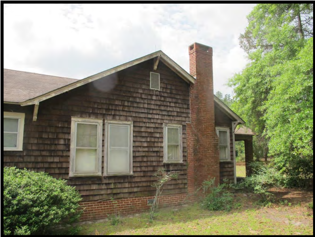
Figure 17: Sinclair House, Looking Southwest.
