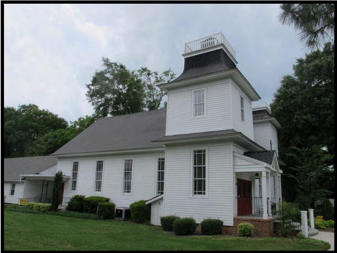
Figure 118: West End Methodist Church, Looking Southwest.
