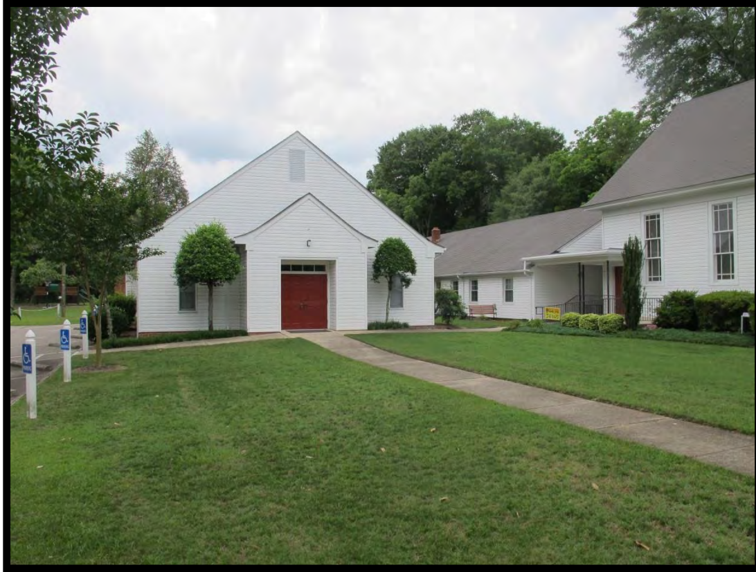
Figure 121: West End Methodist Church, Youth Building Addition, Looking Southwest.
