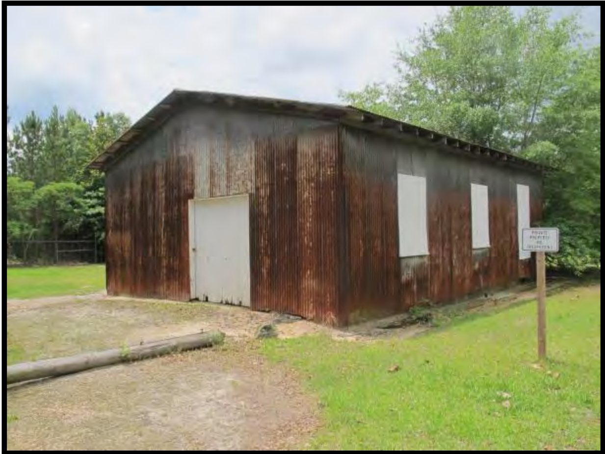
Figure 110: Moses C. McDonald House, Storage Building, Looking Southwest.
