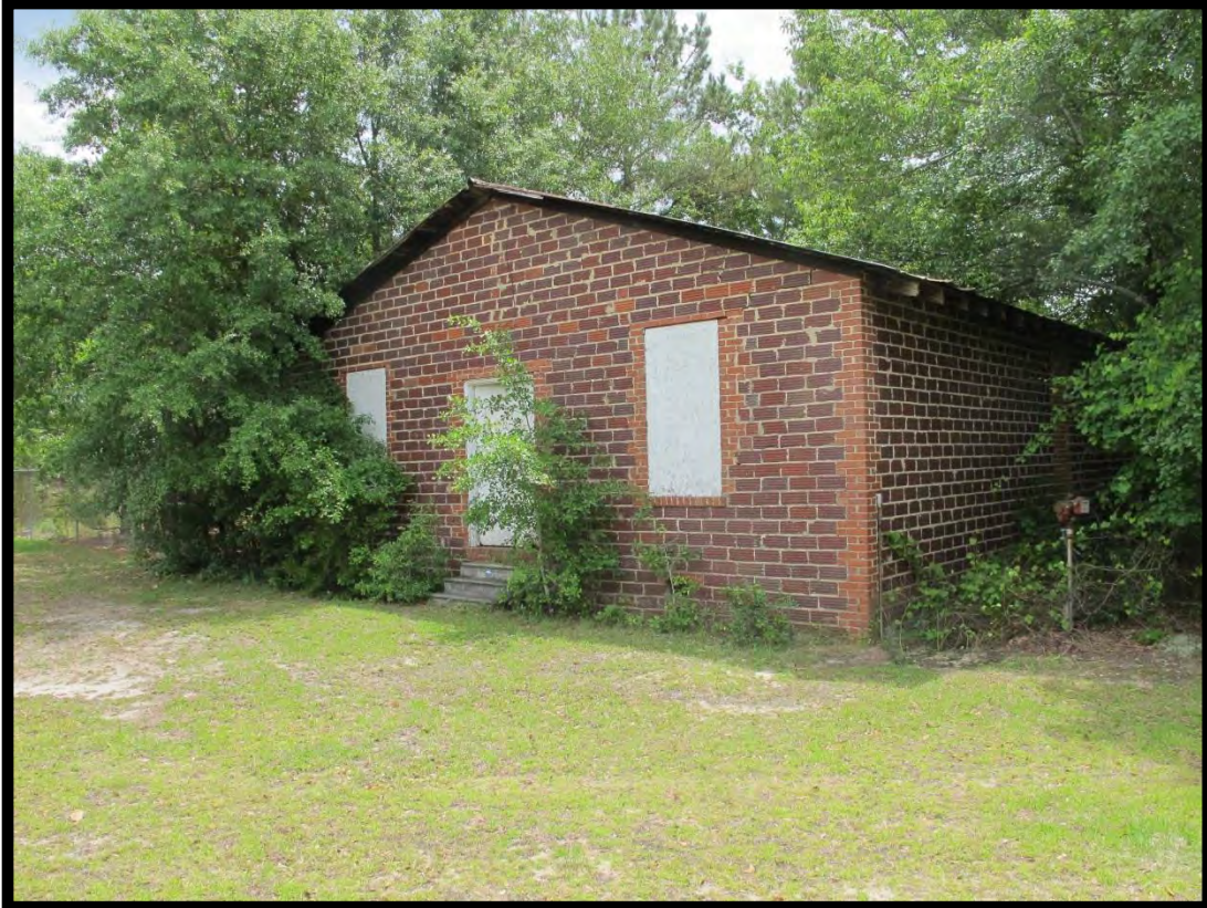
Figure 106: Moses C. McDonald House, Storage Building, Looking Southeast.
