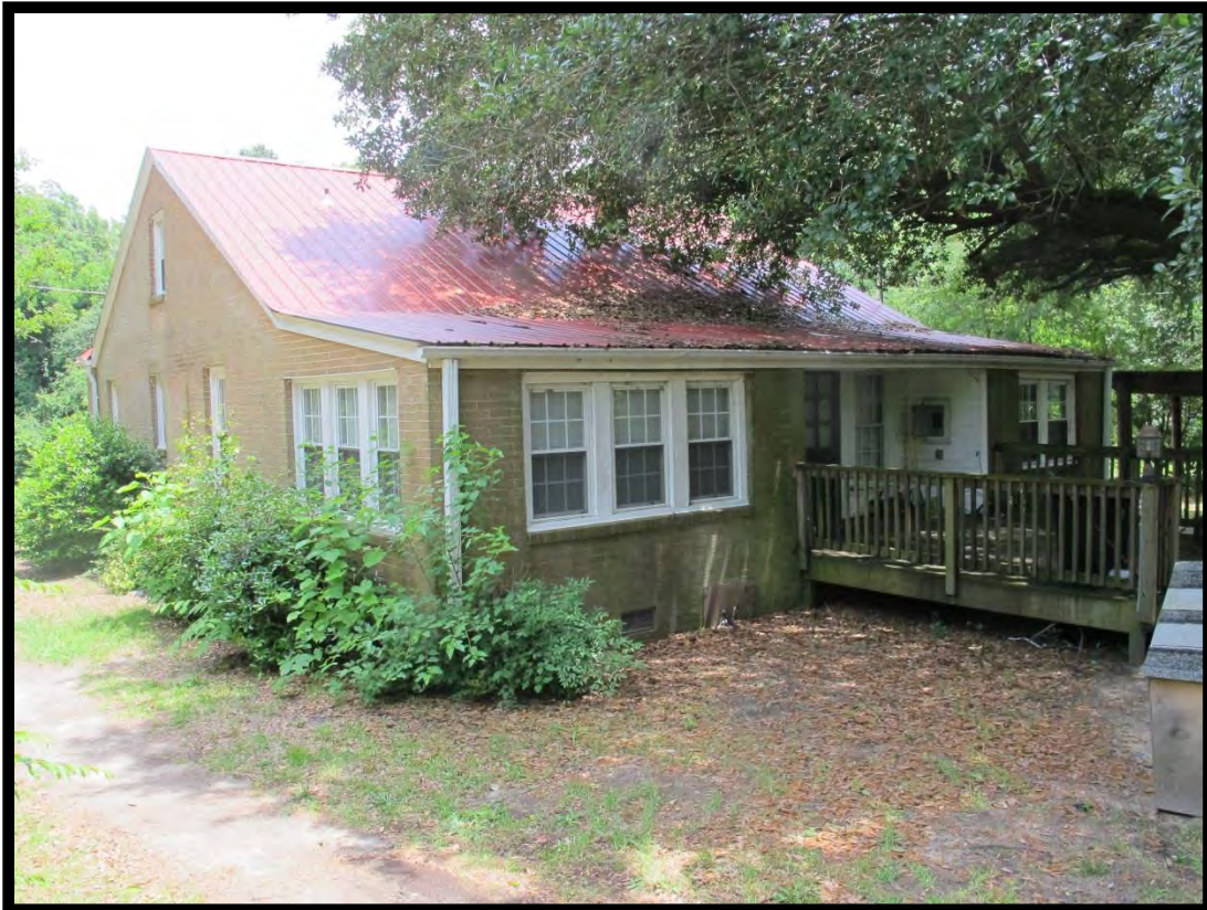
Figure 62: House, Looking Southeast.
