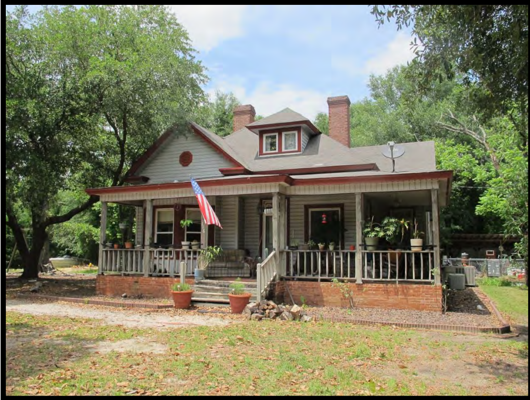
Figure 65: Fletcher House, Looking Northwest.
