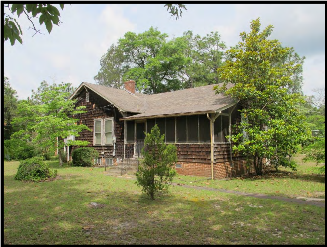
Figure 16: Sinclair House, Looking Northwest.
