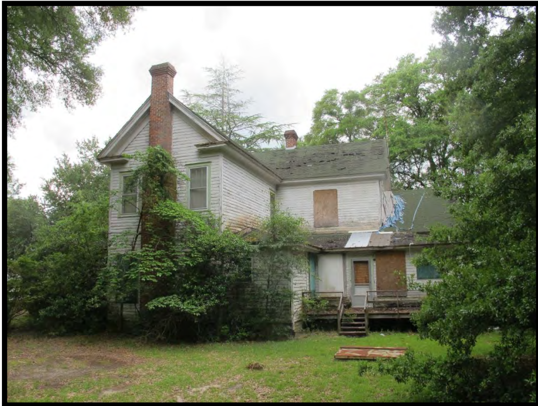
Figure 49: Ritter House, Looking Southwest.
