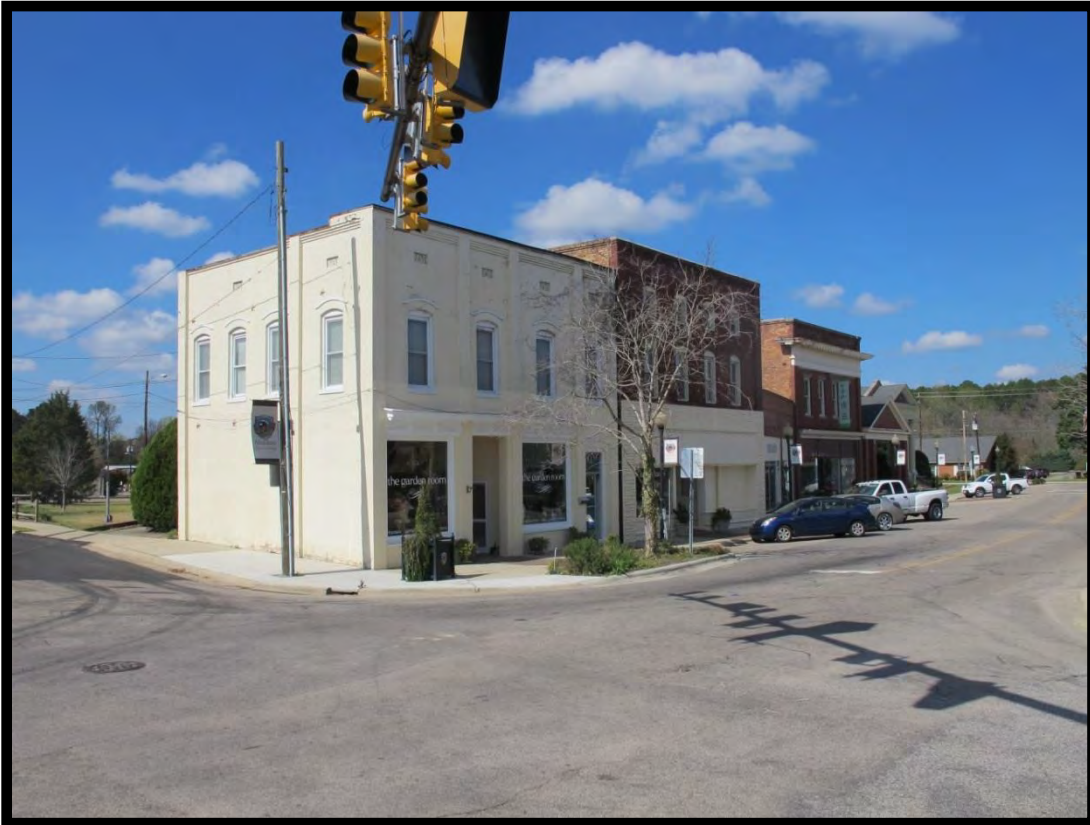
Figure 113: Eva Page Building (MR0099) and Keith Building (MR0100), Looking South.
