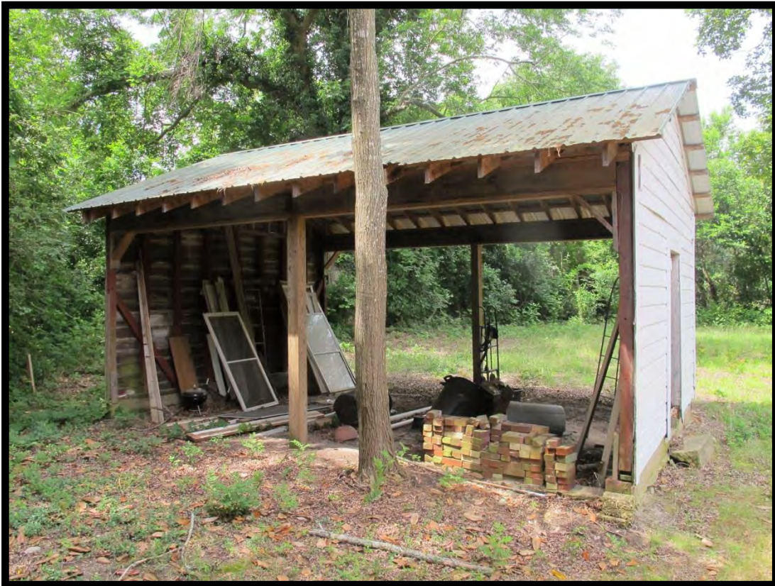
Figure 38: J. B. Von Canon House, Outbuilding, Looking Southwest.
