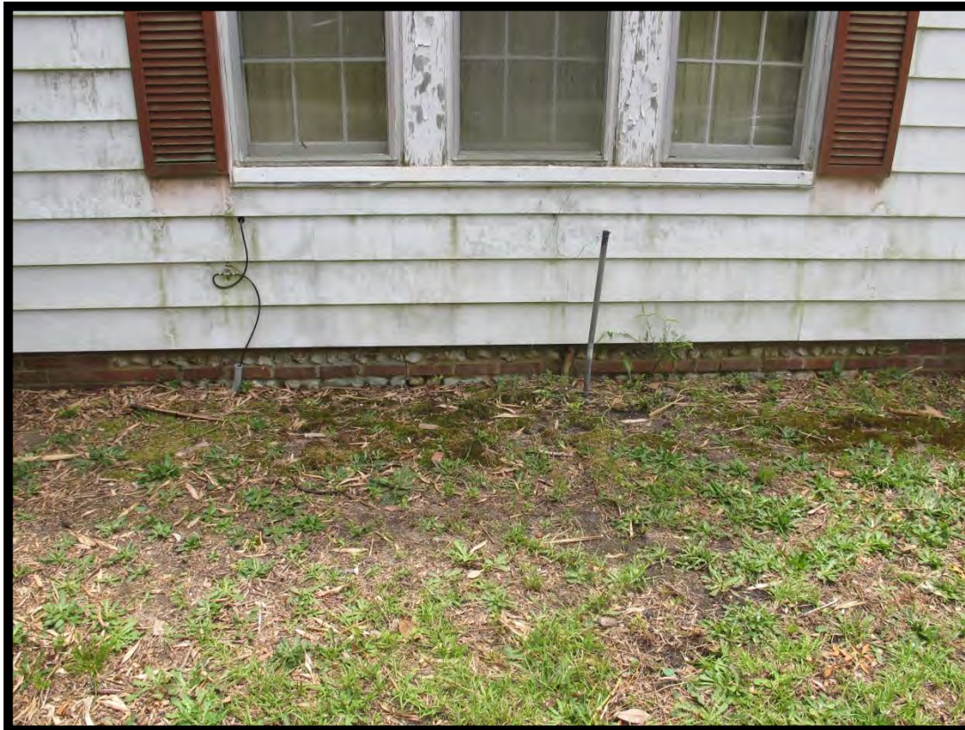
Figure 53: Sutphin House, Detail of Foundation.
