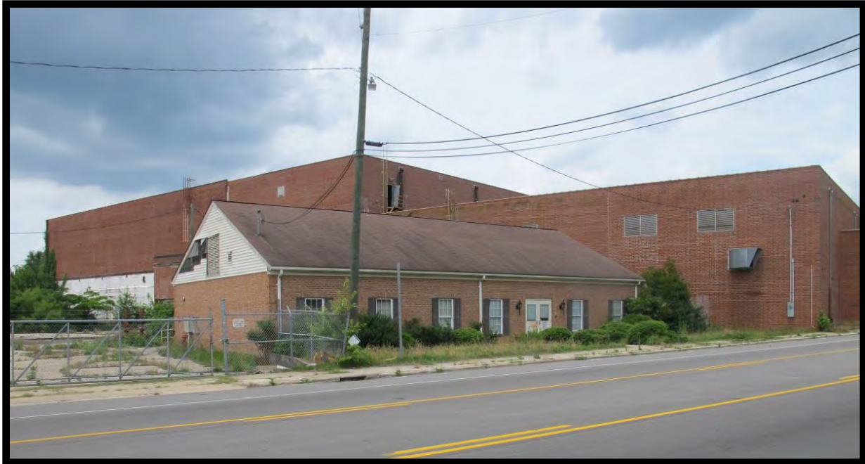
Figure 84: Sandhill Furniture Company, Office Building and Warehouse Looking Northwest.
