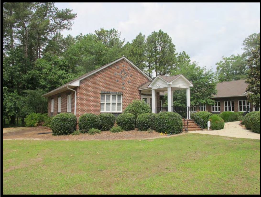
Figure 23: West End Presbyterian Church, Classroom & Office Wing, Looking Northwest.
