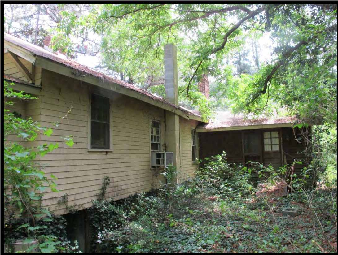
Figure 55: House, Looking Southeast.
