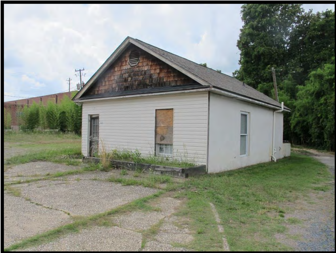
Figure 76: Commercial Block, Former Garage Looking Southwest.
