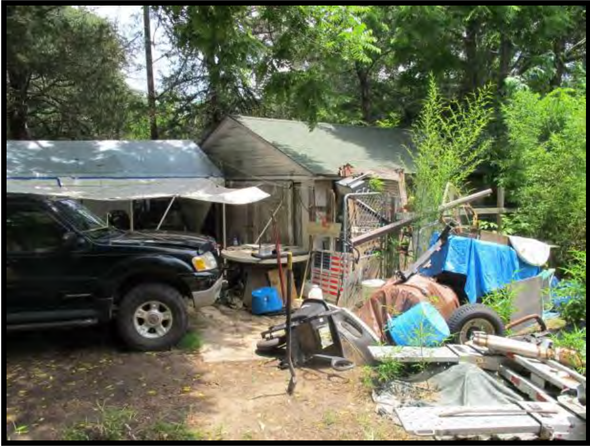
Figure 58: House, Garage Looking Southeast.
