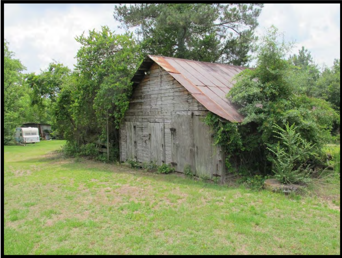
Figure 101: Moses C. McDonald House, Outbuilding, Looking Southeast.
