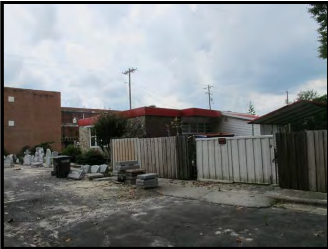
Figure 78: (Former) Carolina Bank, Looking Southwest.
