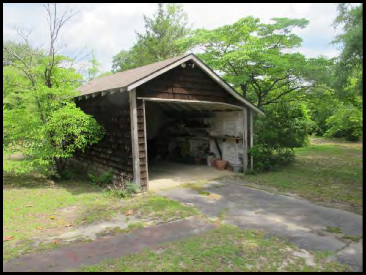
Figure 18: Sinclair House, Garage, Looking Northeast.
