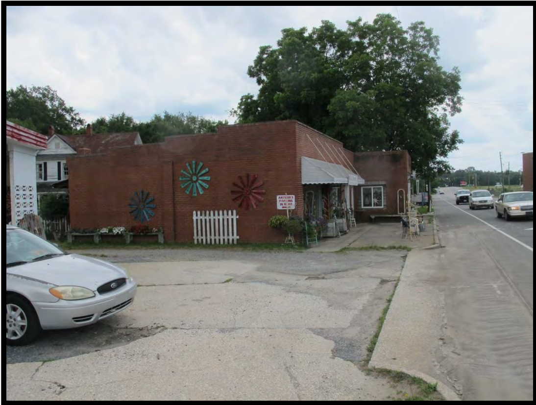
Figure 90: Commercial Block, View of 5353 Looking South.
