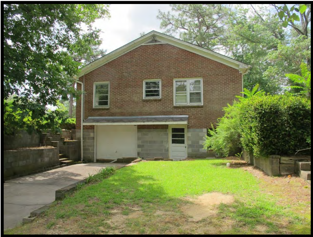
Figure 27: West End Presbyterian Church, Manse, Looking South.
