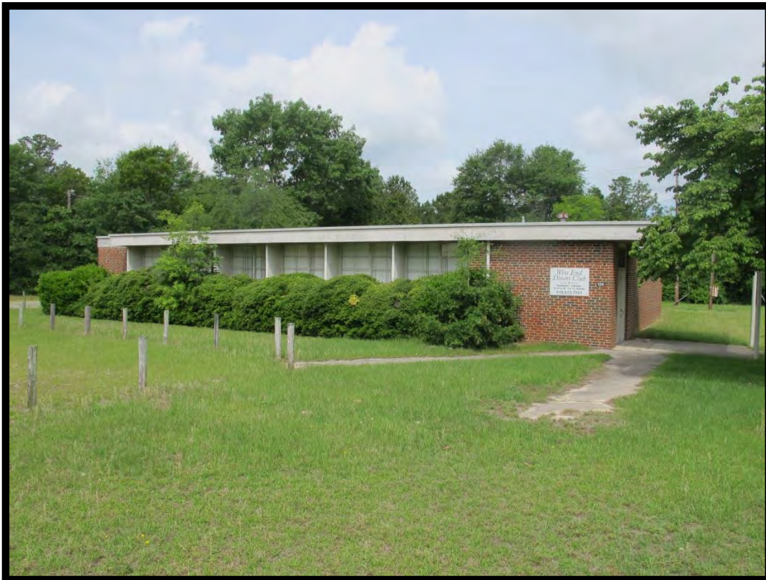
Figure 12: West End High School, Ancillary Building Looking Northwest.
