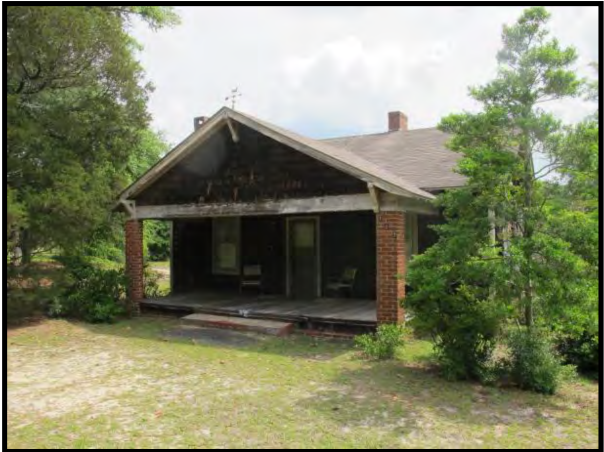
Figure 15: Sinclair House, Looking Northeast.
