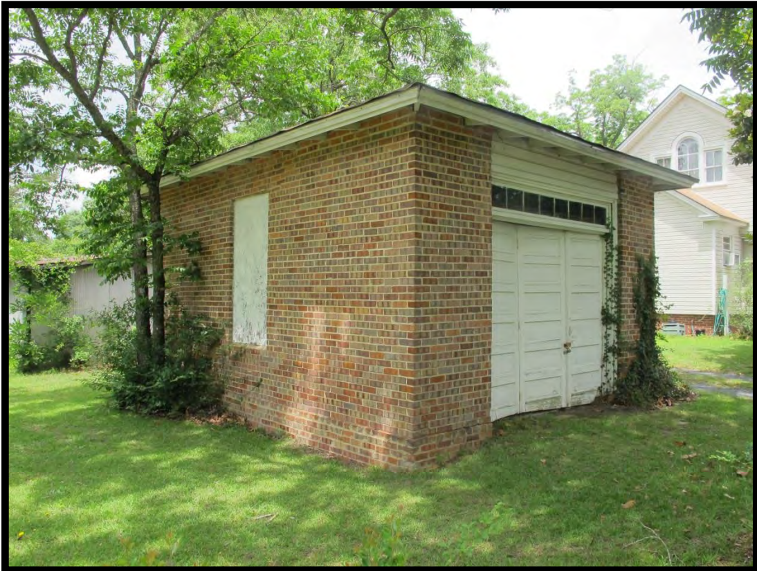
Figure 102: Moses C. McDonald House, Garage, Looking Northwest.
