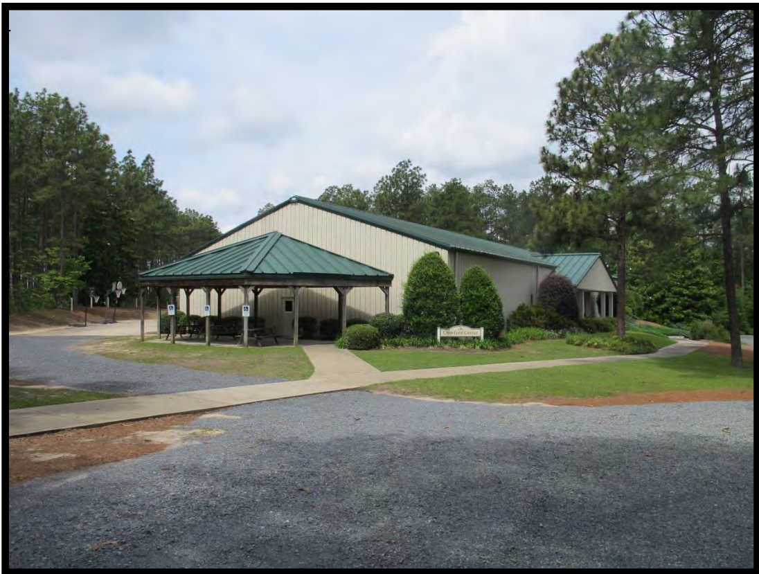
Figure 28: West End Presbyterian Church, Activity Center, Looking Northwest.
