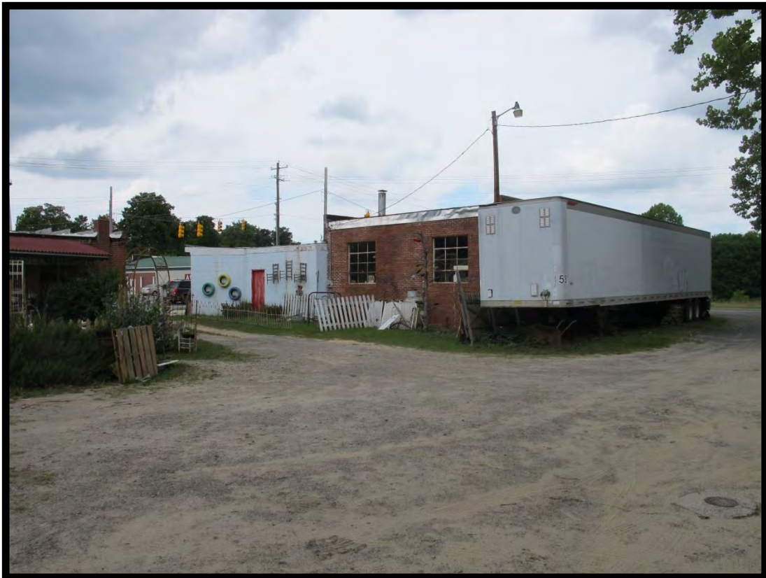
Figure 93: Lewis' Filling Station, Looking Northwest.
