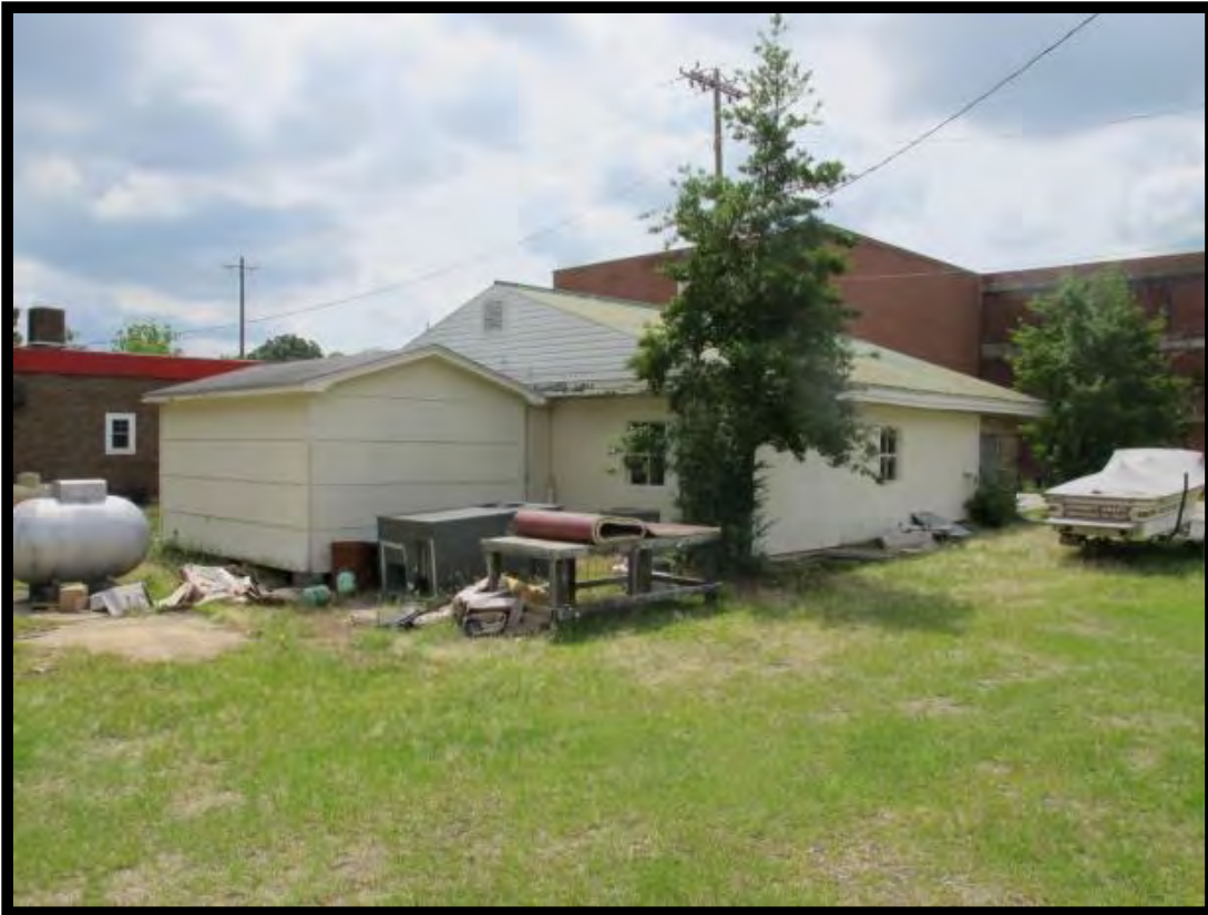
Figure 80: Commercial Building, Looking Southeast.
