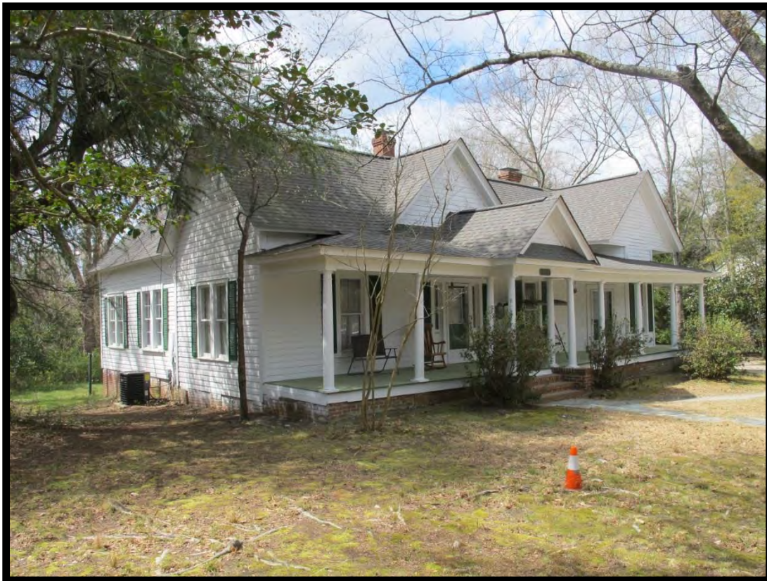
Figure 112: Graham-Thompson House (MR0092), Looking Southwest.
