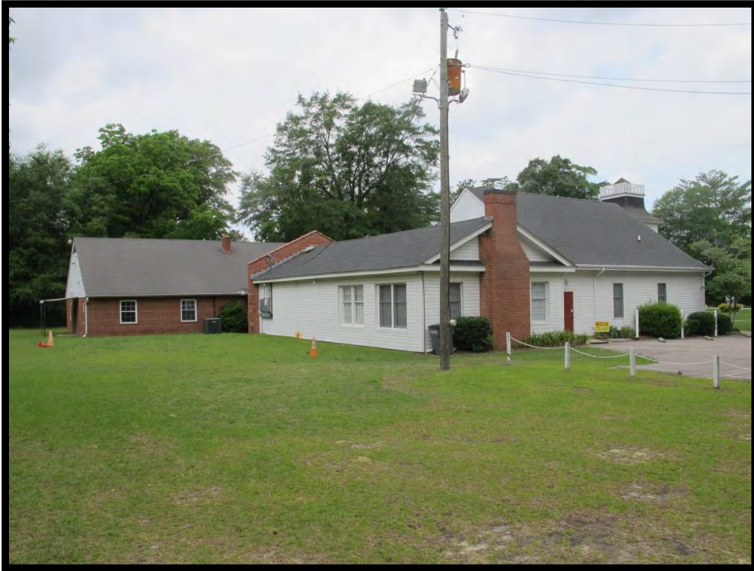
Figure 120: West End Methodist Church, Youth Building, Looking Northeast.
