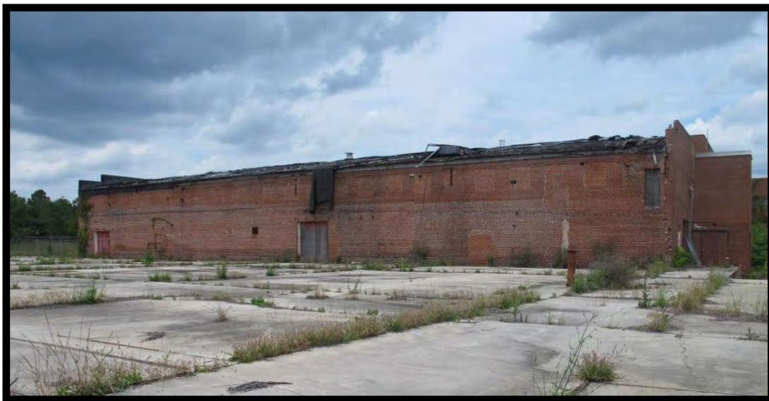
Figure 83: Sandhill Furniture Company, Oldest Factory Building, Looking Northwest.
