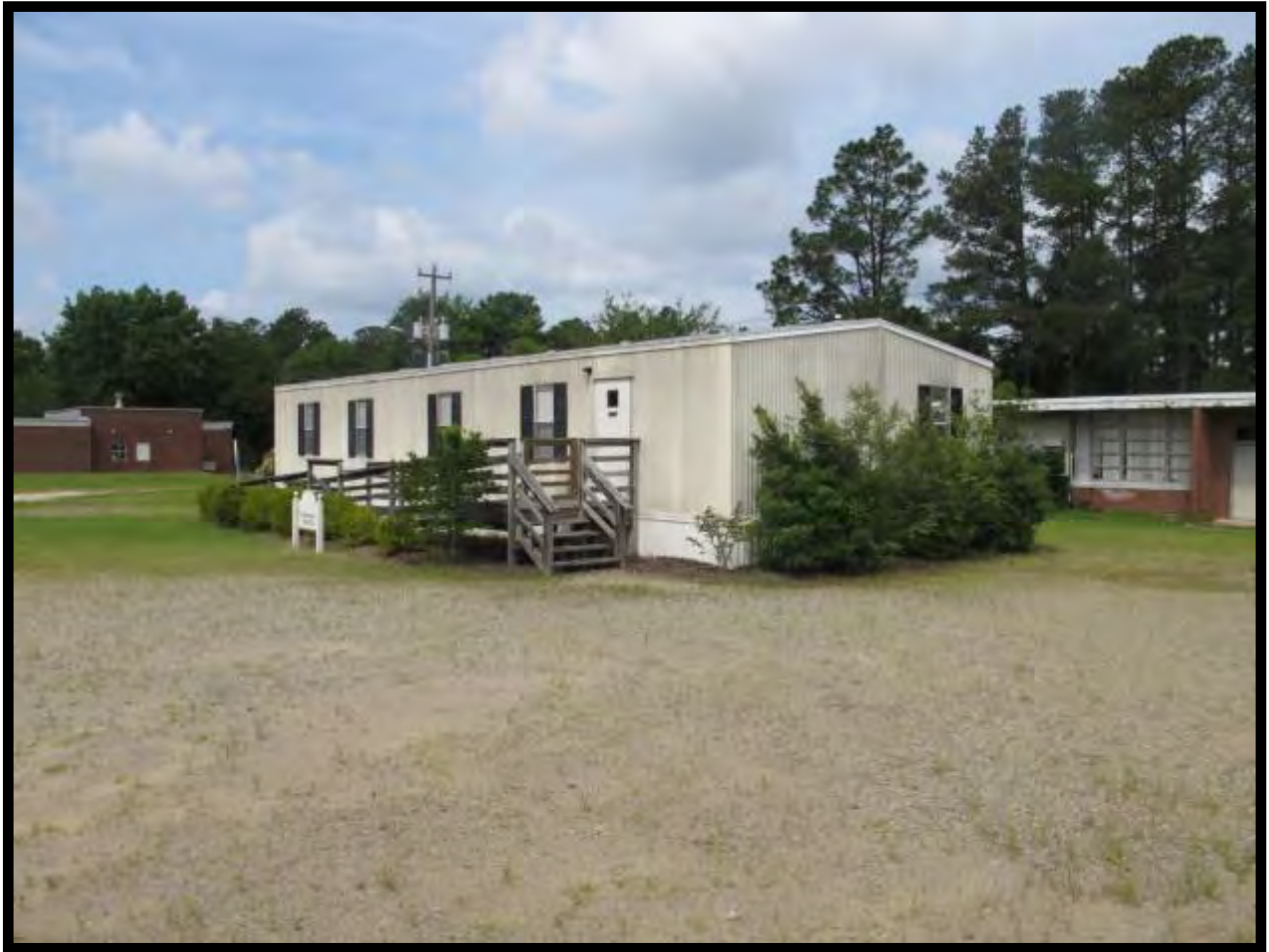
Figure 13: West End High School, Modular Office Looking Northwest.
