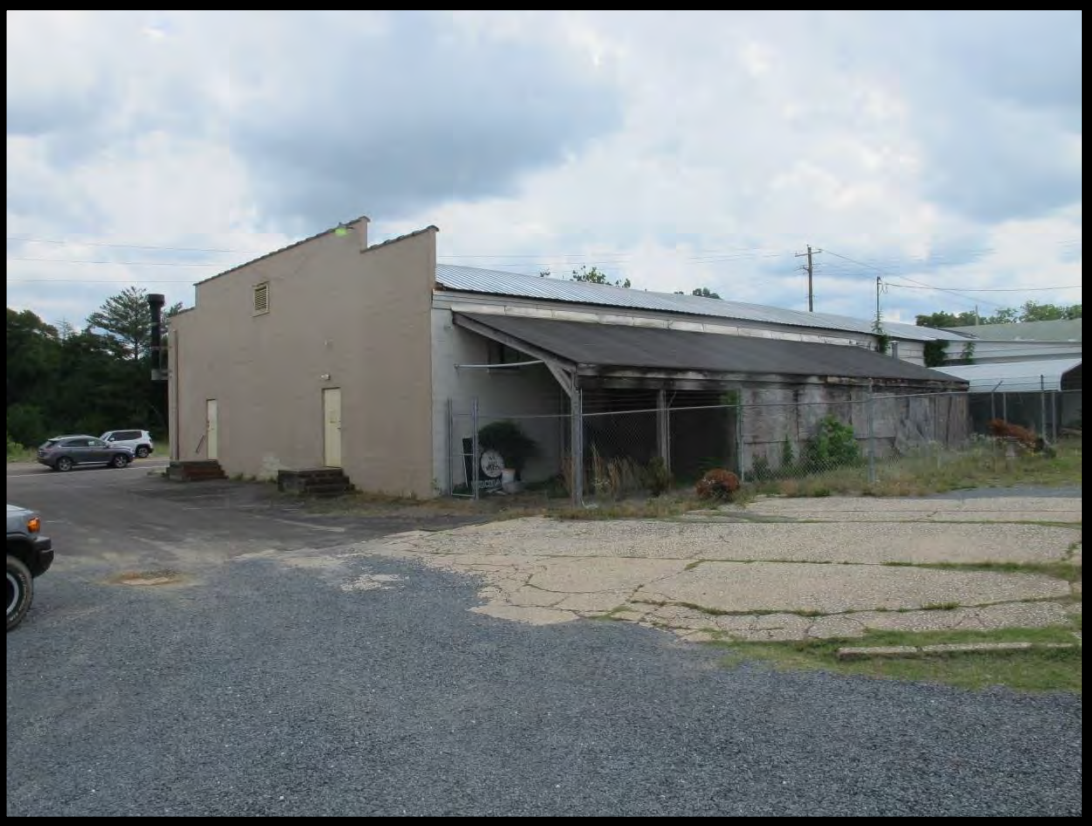
Figure 74: Commercial Block (5326), Looking Southeast.
