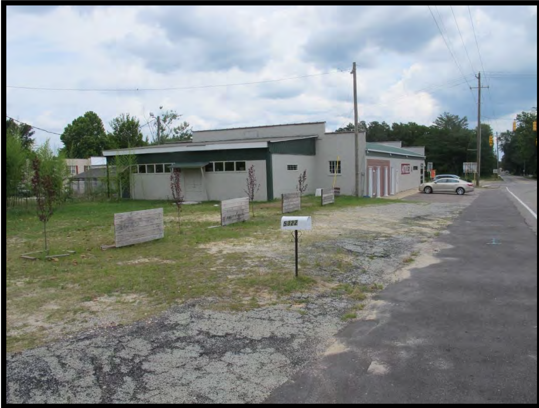
Figure 75: Commercial Block (5336), Looking Northeast.
