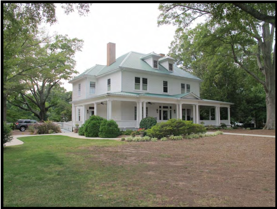
Figure 139: Ransom House (MK1351), Looking Northwest.
