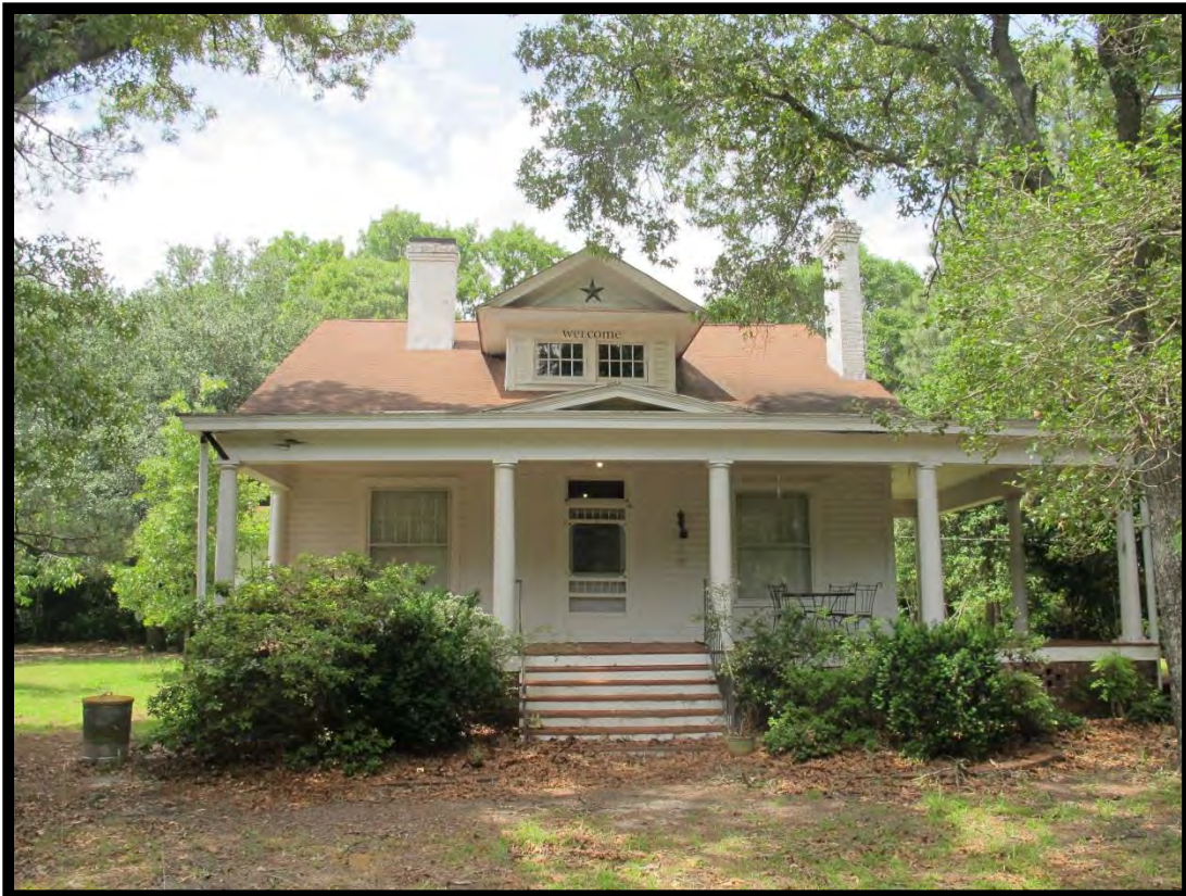
Figure 68: Wilson-Cochran House, Looking Northwest.
