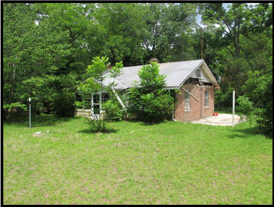
Figure 33: House, Looking Northwest.
