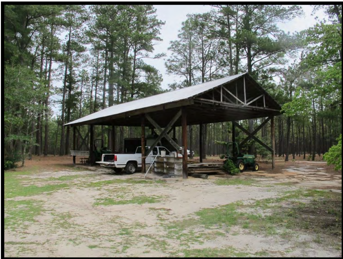
Figure 136: John & Mary Monroe House, Pole Barn Looking North.
