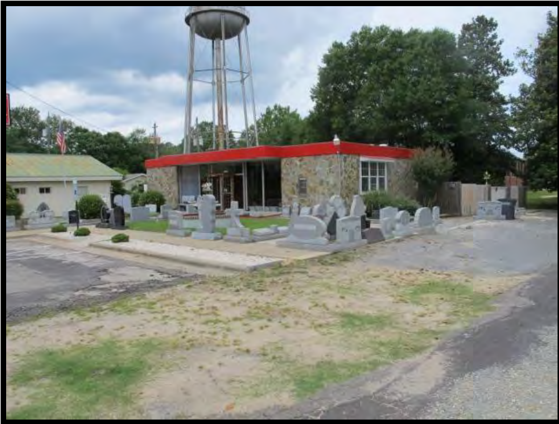
Figure 77: (Former) Carolina Bank, Looking Northwest.
