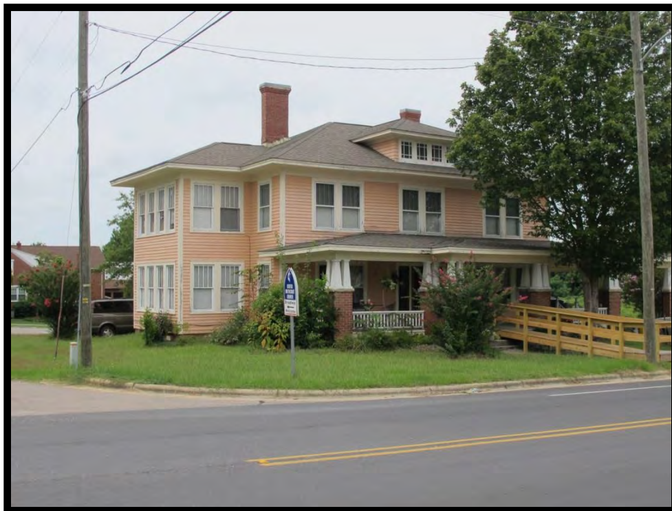
Figure 138: George T. Chandler House (LE0821), Looking Northwest.
