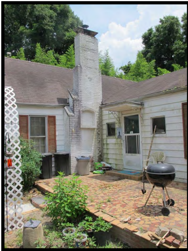
Figure 52: Sutphin House, Detail of Chimney.
