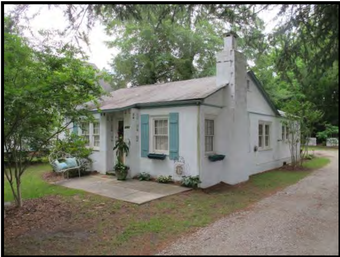
Figure 45: House, Looking Southeast.
