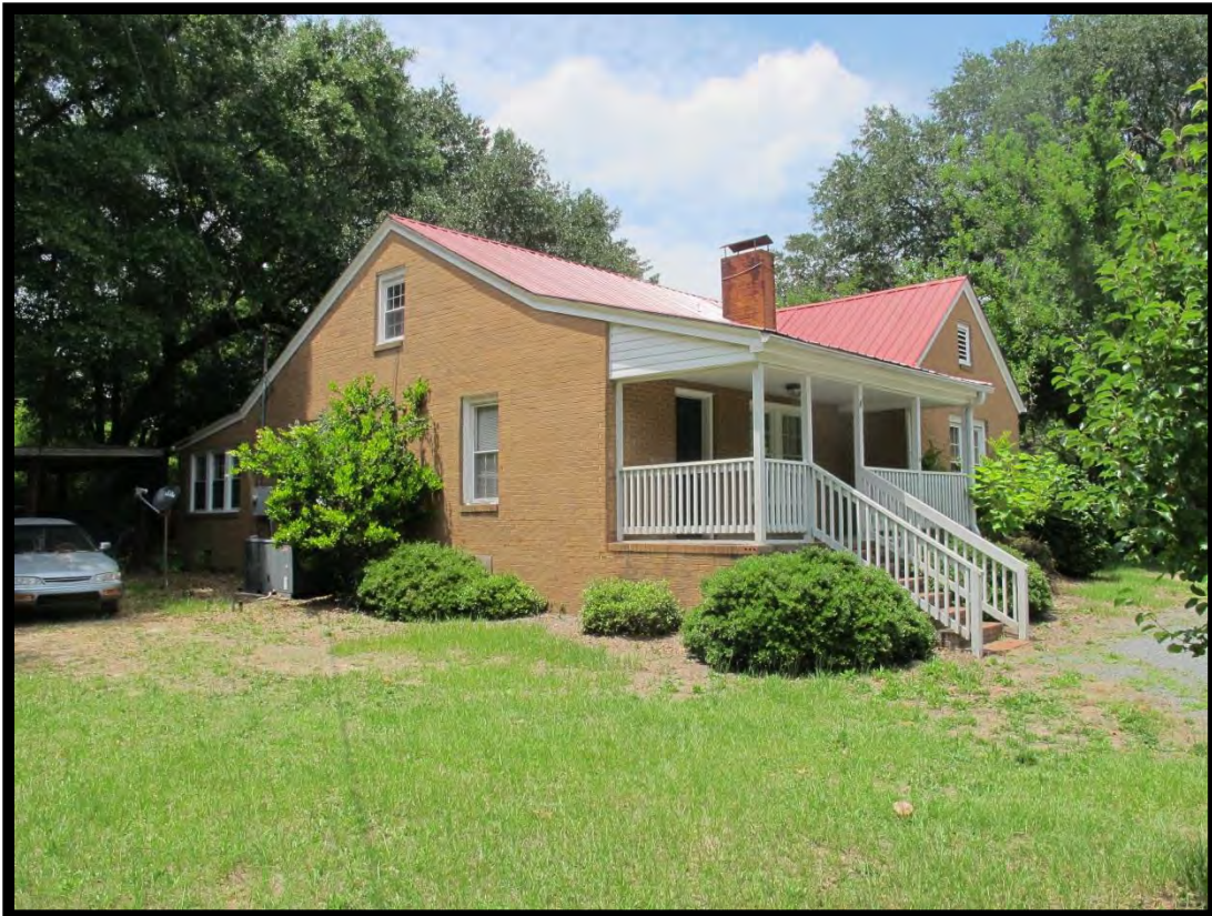
Figure 61: House, Looking Northwest.
