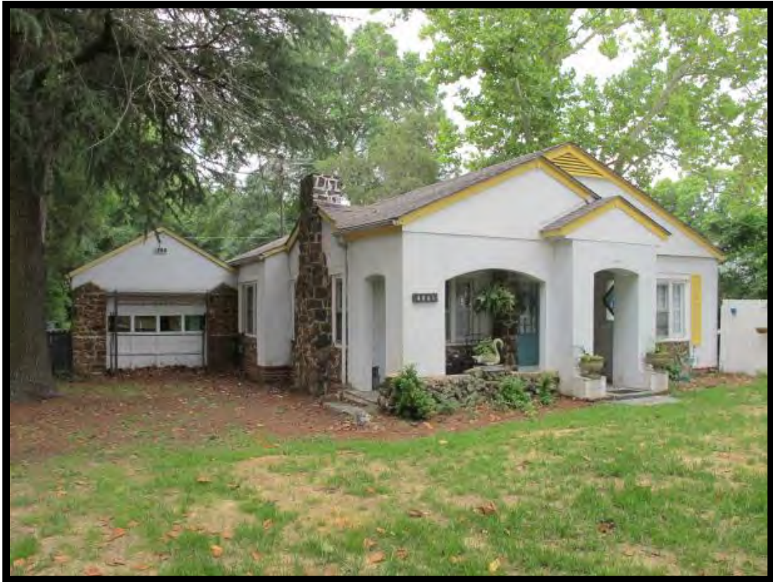
Figure 42: Tucker House, Looking Southwest.
