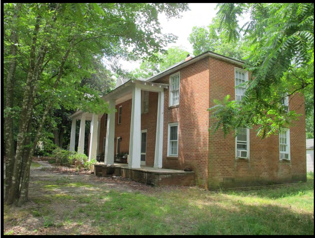
Figure 35: J. B. Von Canon House, Looking Southwest.
