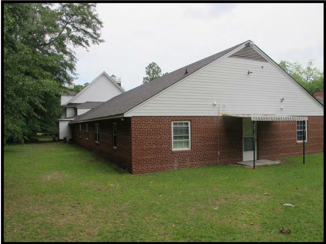
Figure 119: West End Methodist Church, Education Building, Looking Northeast.
