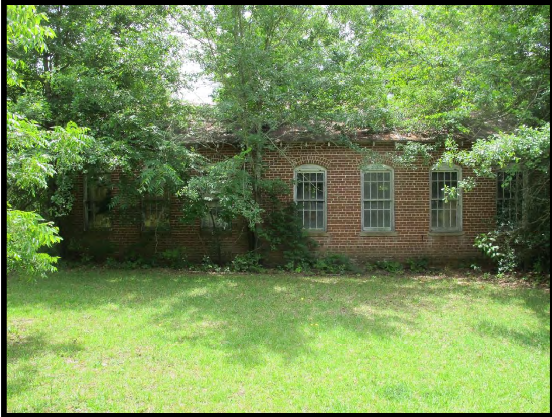
Figure 104: Moses C. McDonald House, Handkerchief Factory, Looking South.
