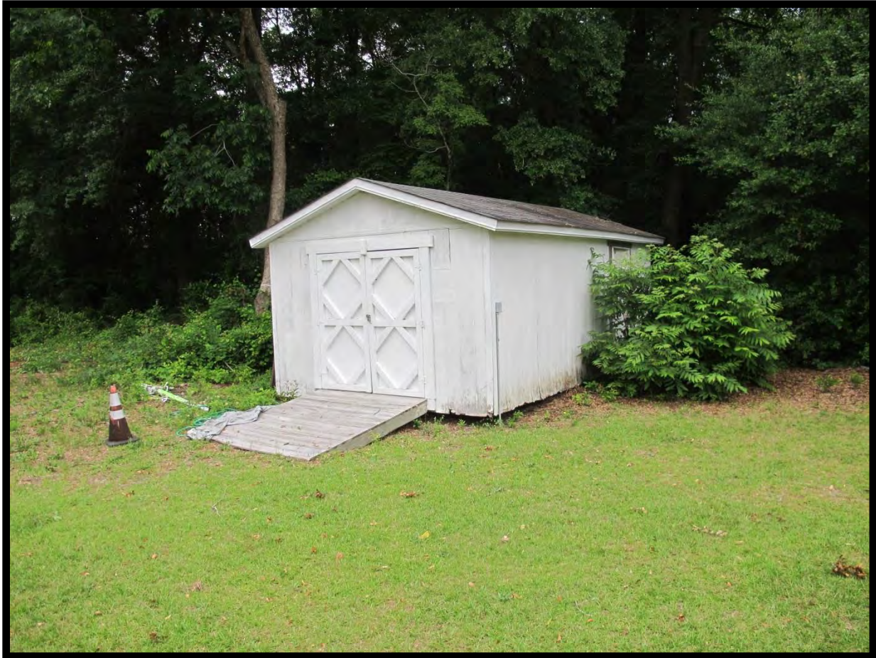
Figure 124: West End Methodist Church, Garden Shed, Looking Southwest.
