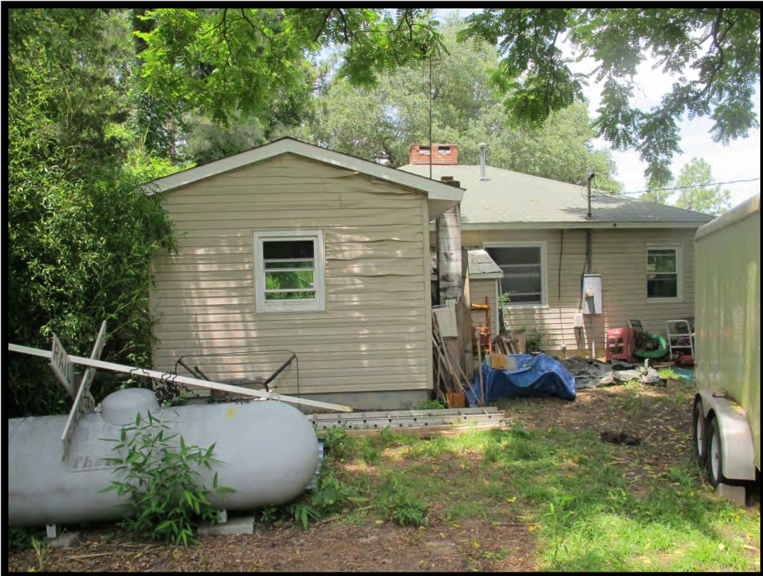
Figure 57: House, Looking Northwest.
